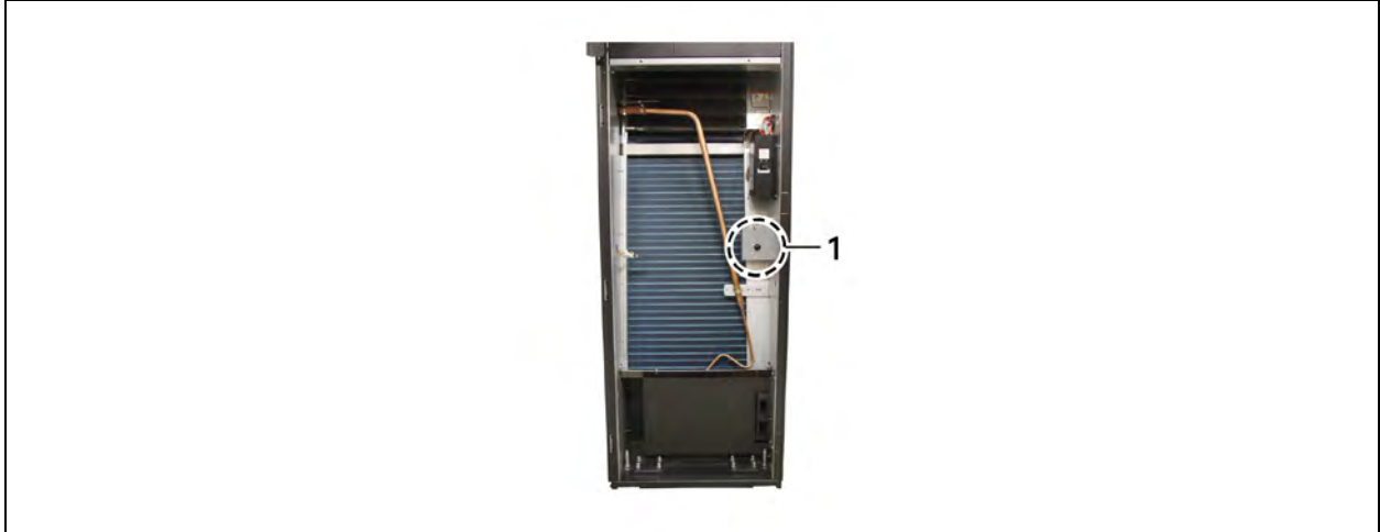
Figure 7.4 Electrical Heating with Temperature Sensor Protection
