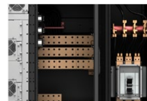
Convenient jumpers allow for single or dual input connections.
