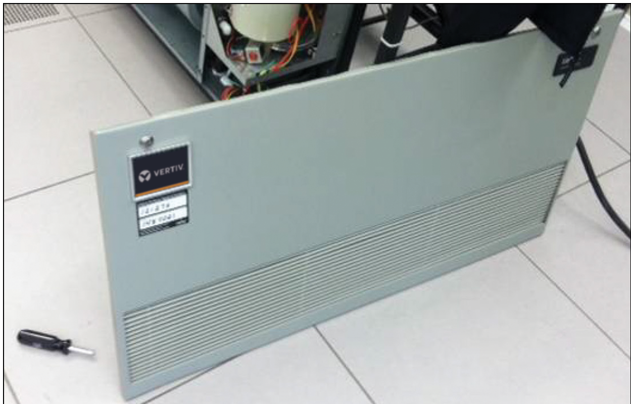
Figure 7.21 Remove DME evaporator front access cover
