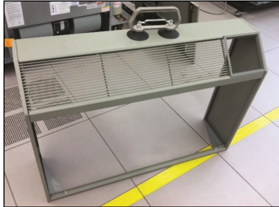
Figure 7.23 Remove evaporator panel assembly
