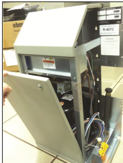
Figure 7.27 Remove front access cover from condensing unit
