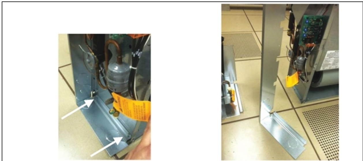
Figure 7.24 Remove left chassis extension
