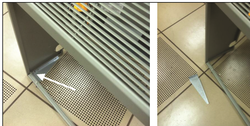
Figure 7.26 Remove bottom left support bracket from DME evaporator panel
