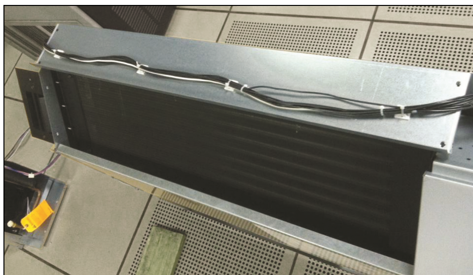
Figure 7.31 Power/control wire harness routing
