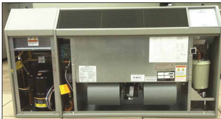
Figure 7.33 Install DME evaporator panel assembly
