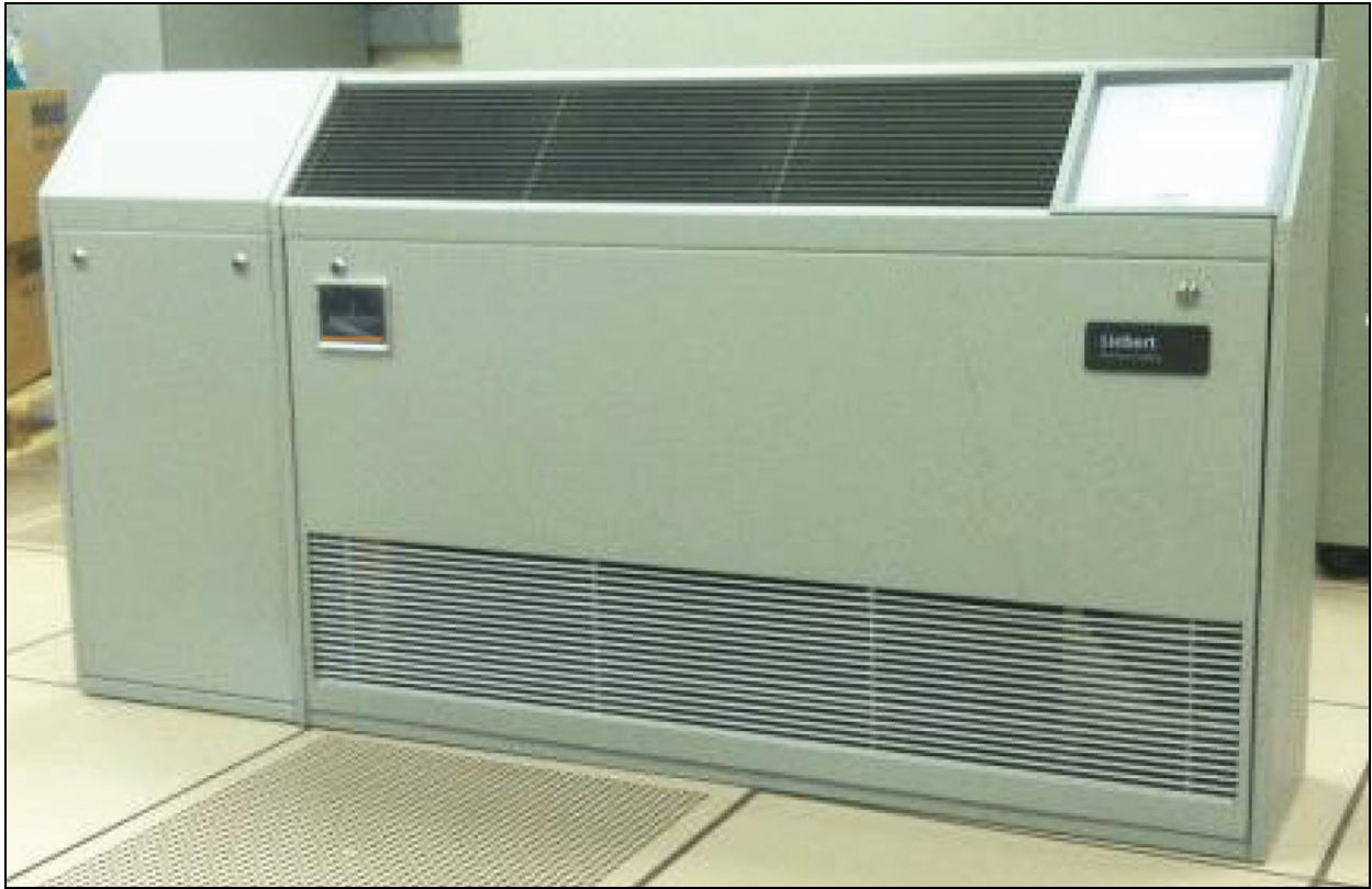
Figure 7.34 Install DME and DMC front access covers
